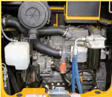
• Engine, filters and coolant reservoir
